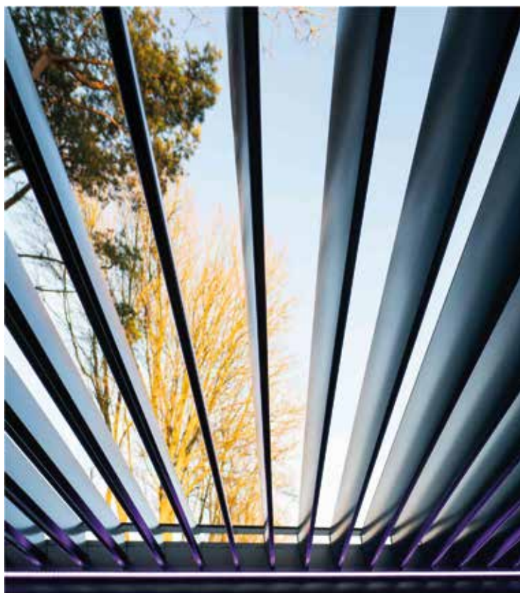
• Roof louvers in open position
